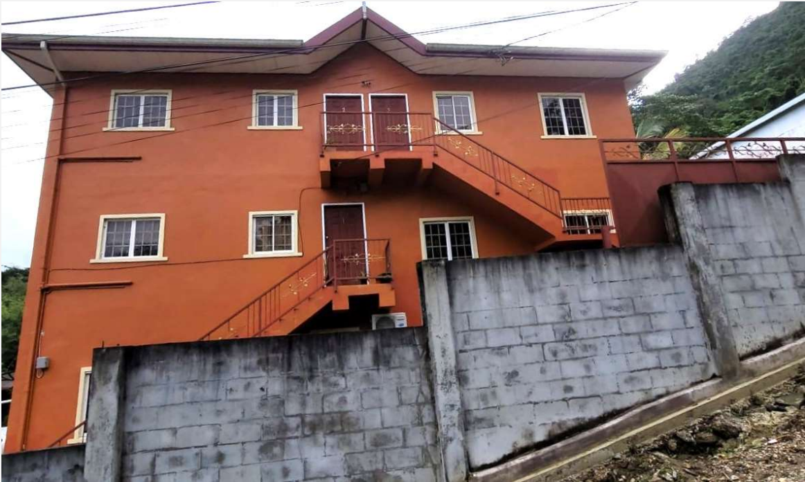
View of Building's Exterior
